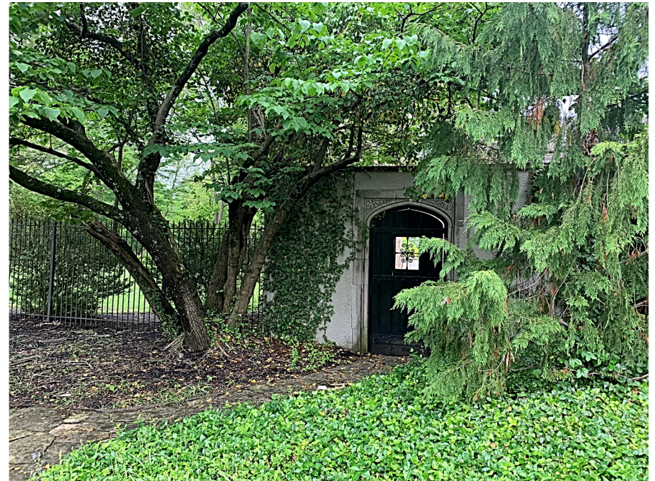
East garden wall & fence
