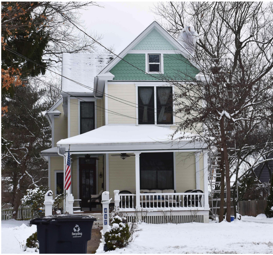
CLAPBOARD SIDING WITH SHAKE SIDING FRONT PORCH
