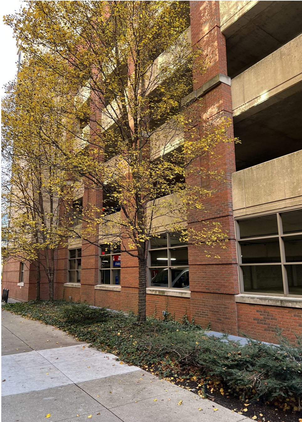
+/-8' bed in a service alley/pedestrian connector (Arena District)
