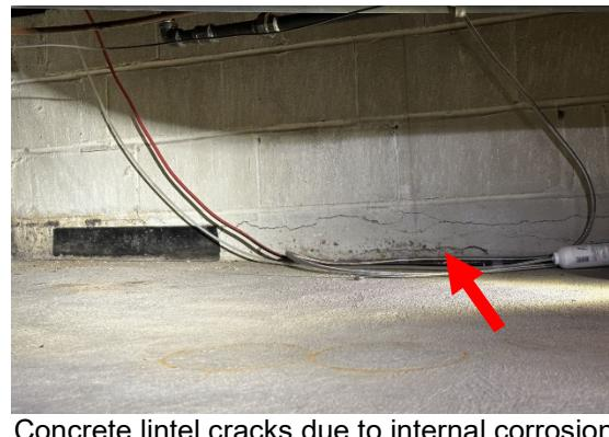
Concrete lintel cracks due to internal corrosion
