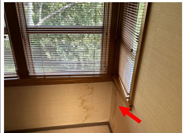
Water infiltration at north side wall / low roof
